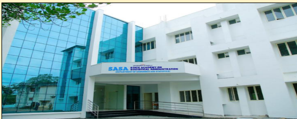
State Academy of Statistical Administration (SASA) building, Kerala
