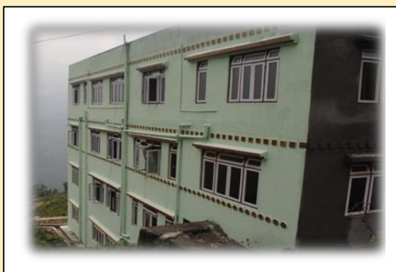
DESM&E Headquarter building at Sokeythang, Gangtok
