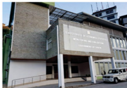
DESM&E Headquarter building, Sikkim
