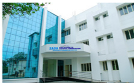
State Academy of Statistical Administration (SASA) building, Kerala
