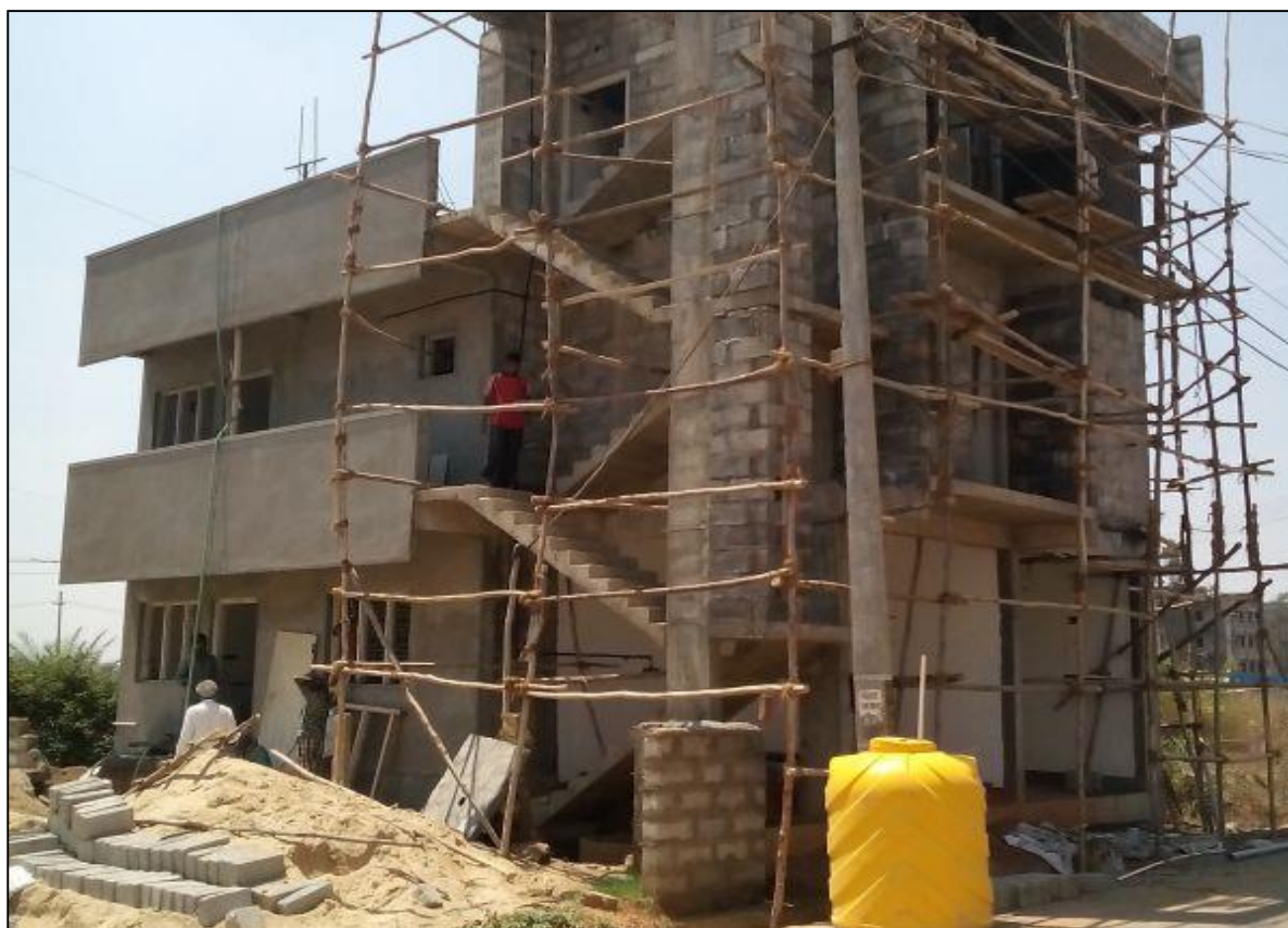
Figure 3.58 Residential building with Cement Concrete blocks under construction
