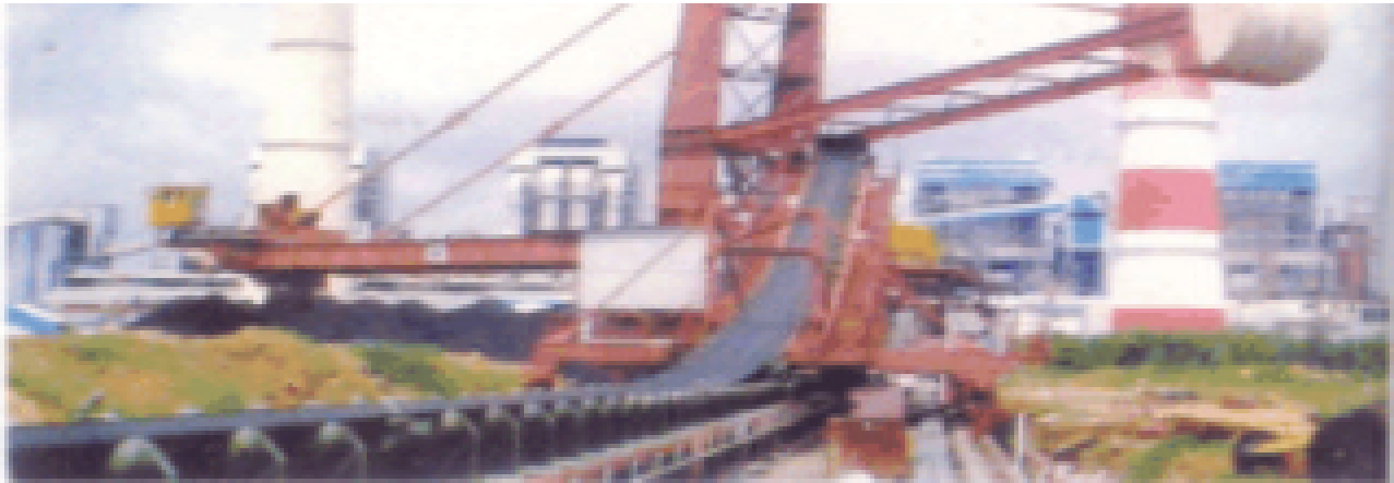
NTPC Talcher Stage-II (4x500MW)- Overall View
