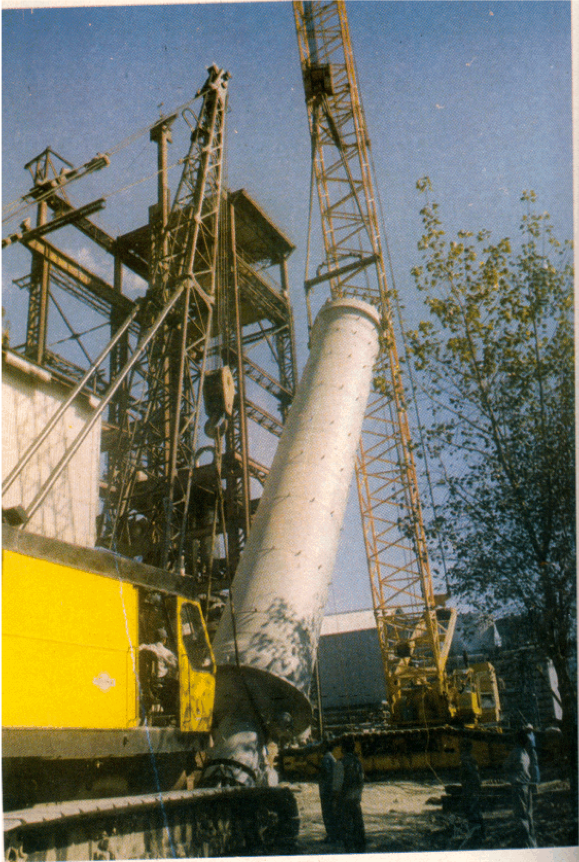
Erection of synthesis converter of ammonia-II plant.
