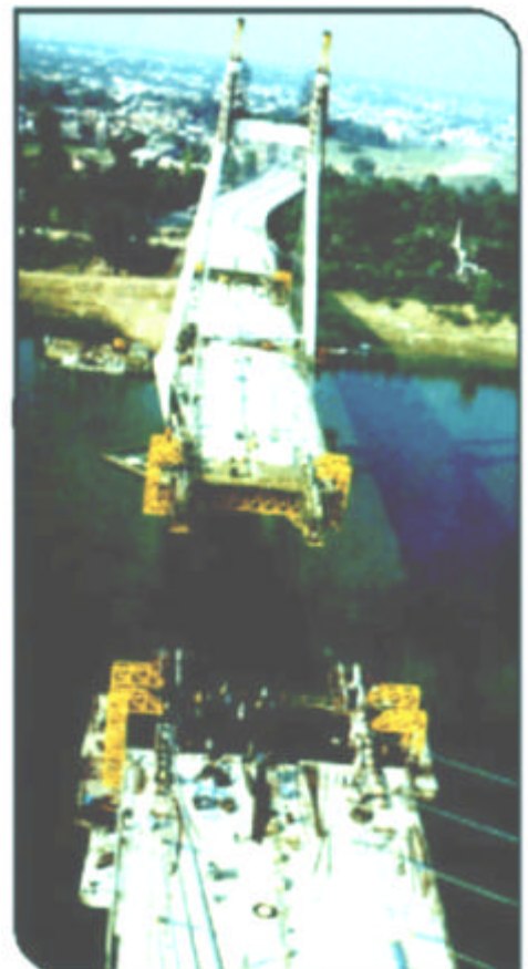
Cable Bridge under construction at Naini (Allahabad)
