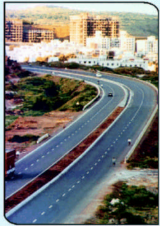
Approaching Pune City on NH-4
