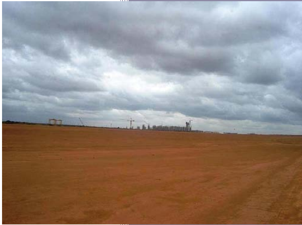
New Bangalore International Airport, India
