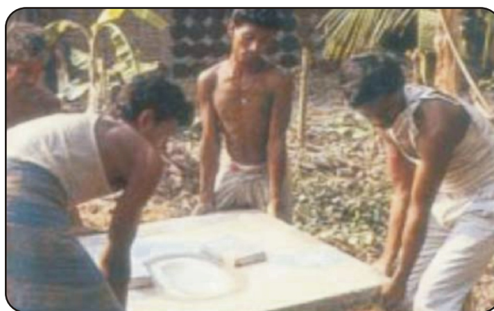
Sanitary pan being laid under Total Sanitation Campaign
