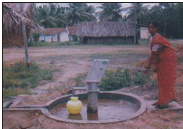
Handpump with platform and drainage
